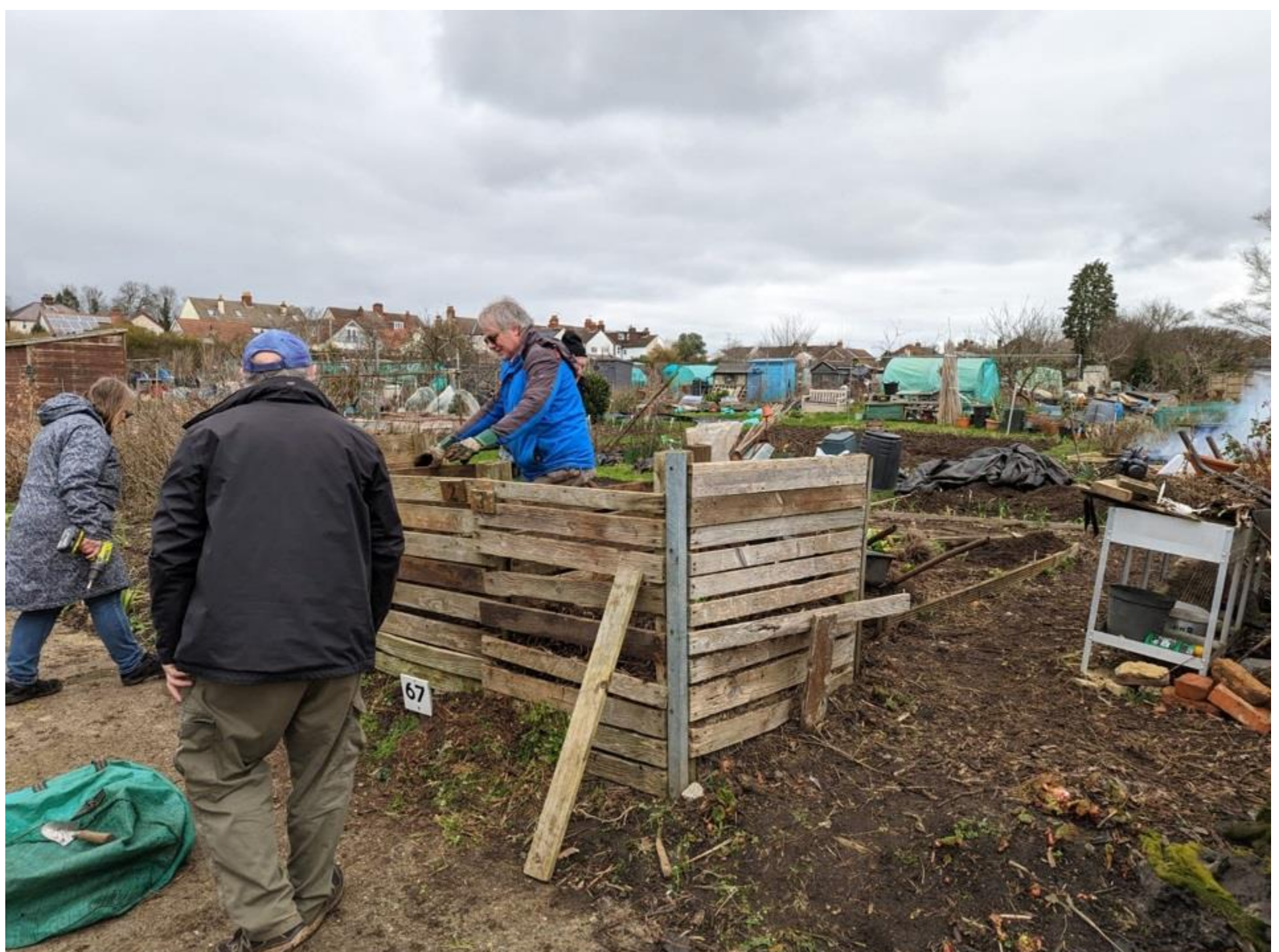
Spring clean at the allotment plus compost bin repairs
