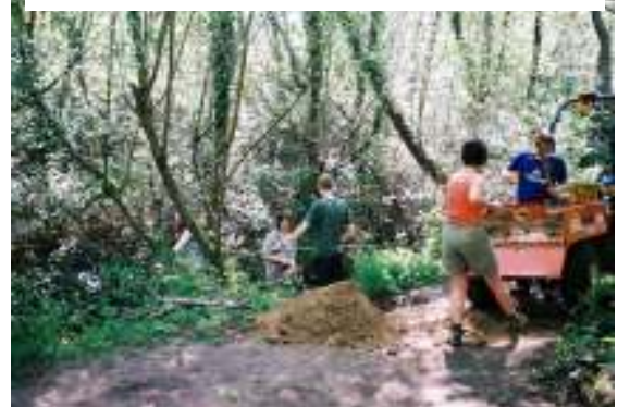
Estate management: Stream bank repairs
